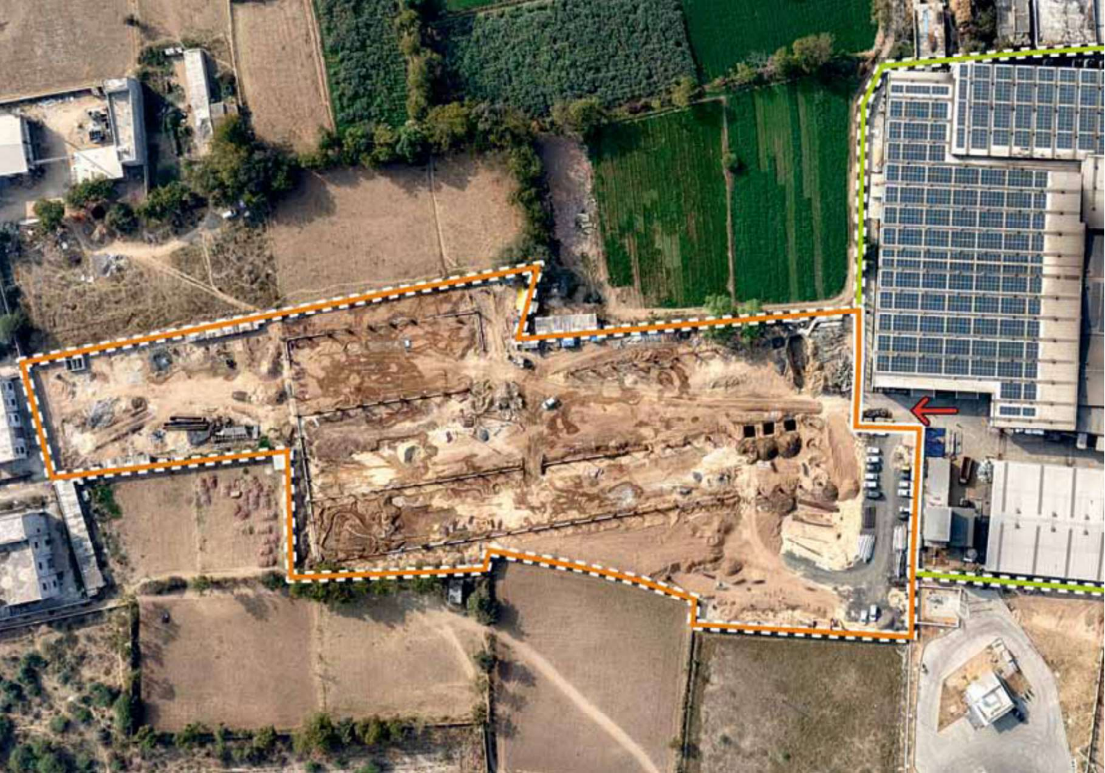
An aerial view of the Scoda Tubes site – outlined is the space for the expansion of seamless pipe production.
